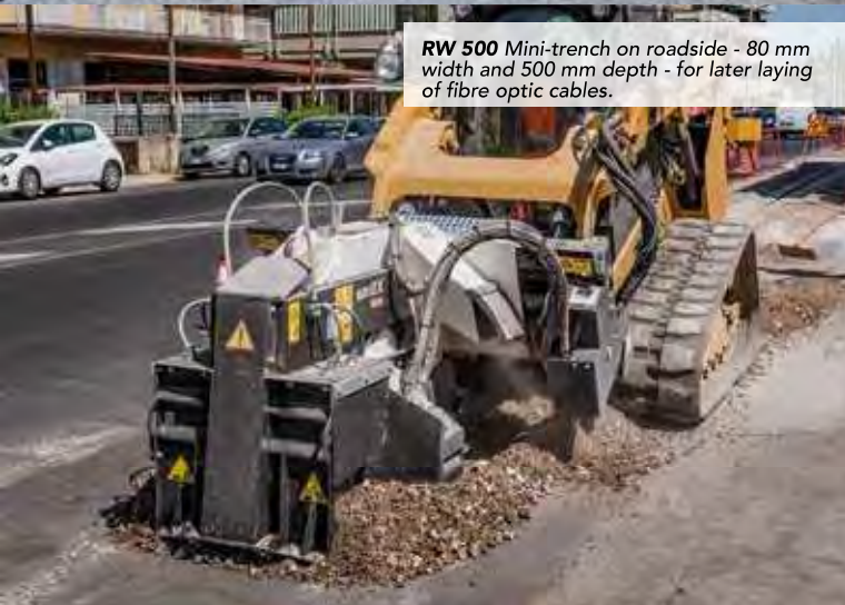
RW 500 Trench at 120 mm width for laying fibre optic cables.
